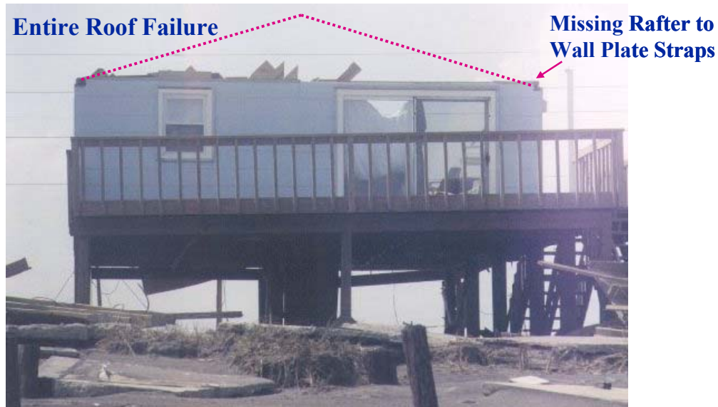
Figure 1-5. Roof Truss/Rafter to Wall Connection
