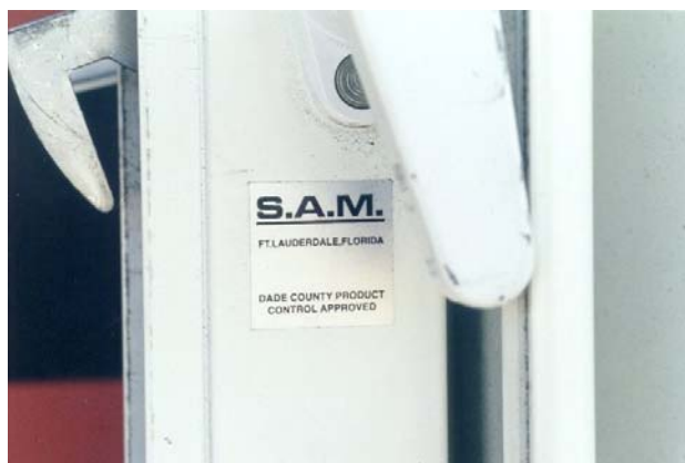
Figure C-9. Two product approval sticker on accordion shutters indicating that they meet Miami-Dade County impact resistance and wind pressure load standards. These labels contain the words “Dade County Product Approved” or equivalent.
