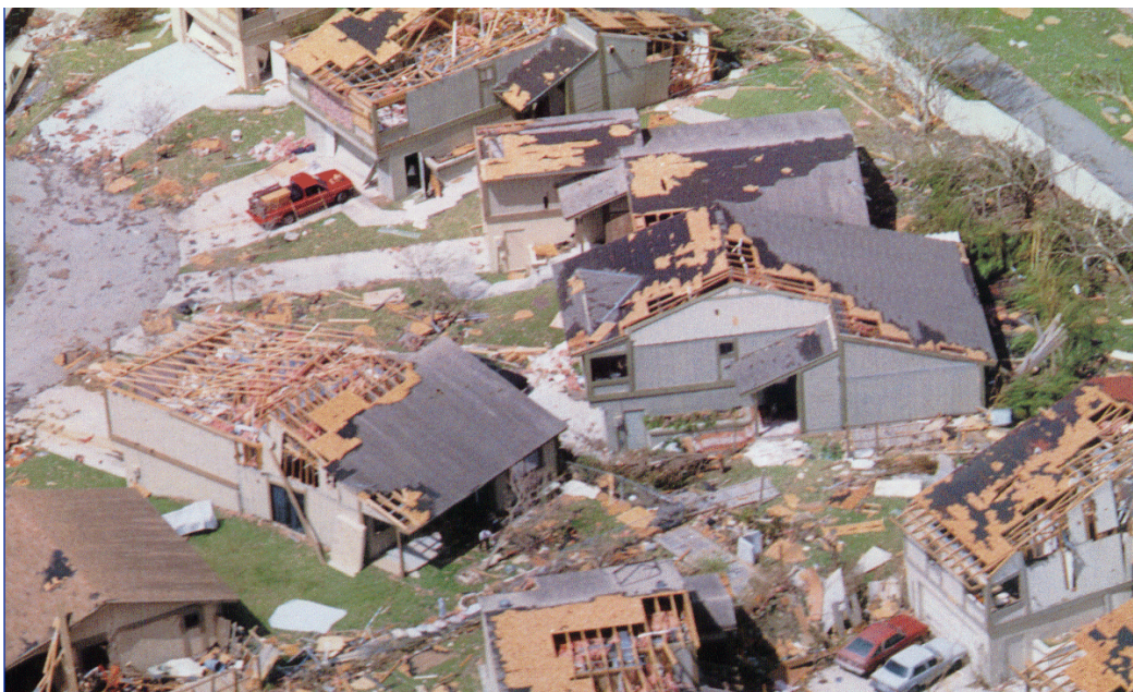
Figure 1-4. Roof Deck Performance
