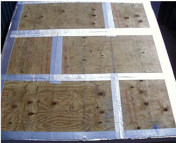
Figure C-1. Self-Adhering Modified Bitumen Strips Applied to Plywood Joints of Roof Deck
