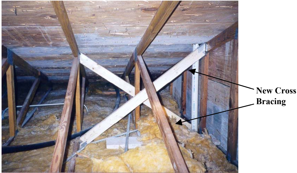
Figure C-8. Gable End Bracing Secured with Metal Connections
